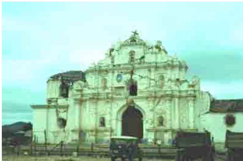
(Figure 10 – Photo of the church in Comalapa alter the 1976 earthquake
